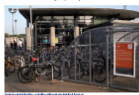
Cycle parking facilities at Ashford International Station
